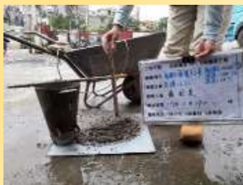
混凝土坍度試驗
