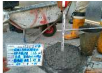
混凝土坍度試驗
